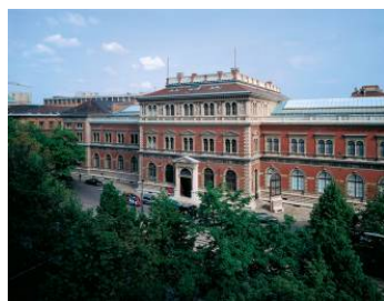
Front view of the MAK façade © Gerald Zugmann
